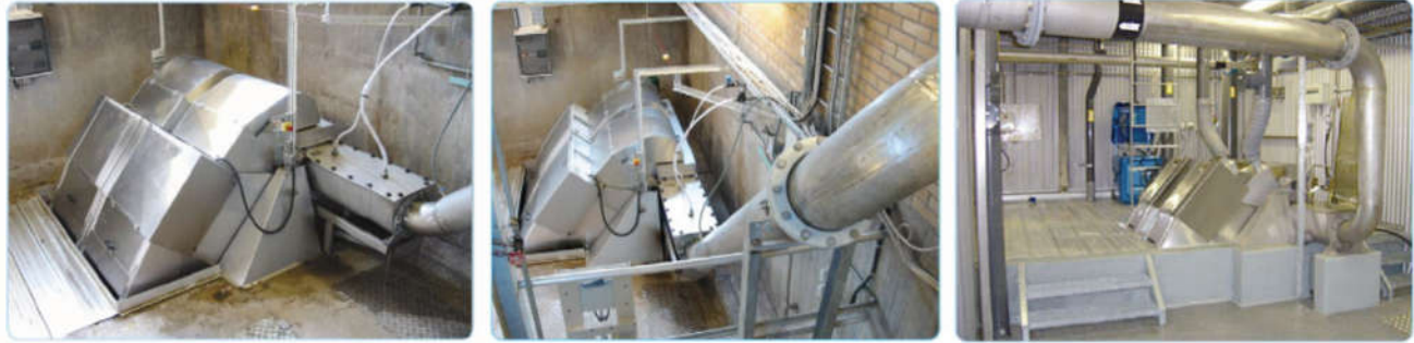
2 Sample Facilities in Sweden with Extended Wash Press Pipe Systems
