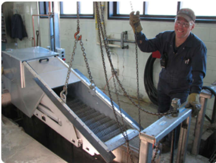
Asbestos WWTP, QC
