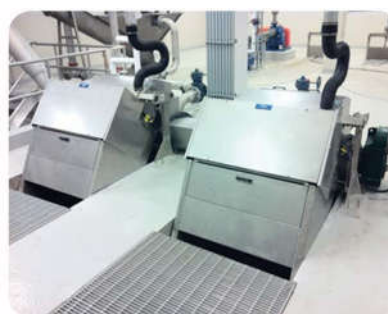
Hawkesbury WWTP, ON (2012)
