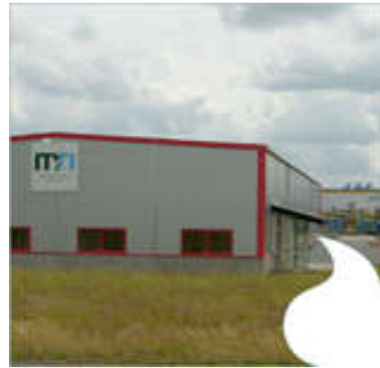
M&N production shop.
