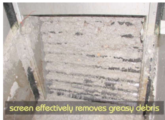
1mm Screen Removing Bacon Processing Grease Without Hot Water Spray Addition
