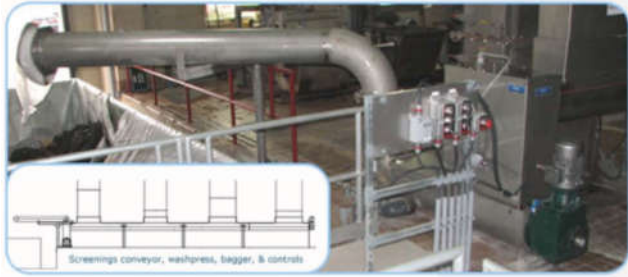
2 Sample Facilities in Sweden with Extended Wash Press Pipe Systems
