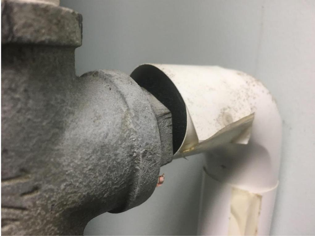
*Figure 31 – Observed black foam insulation around pipe, no need to sample*
