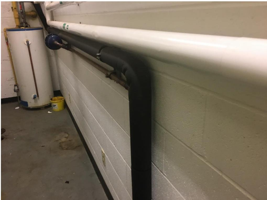
Figure 40 – Observed black foam insulation, no need to sample
