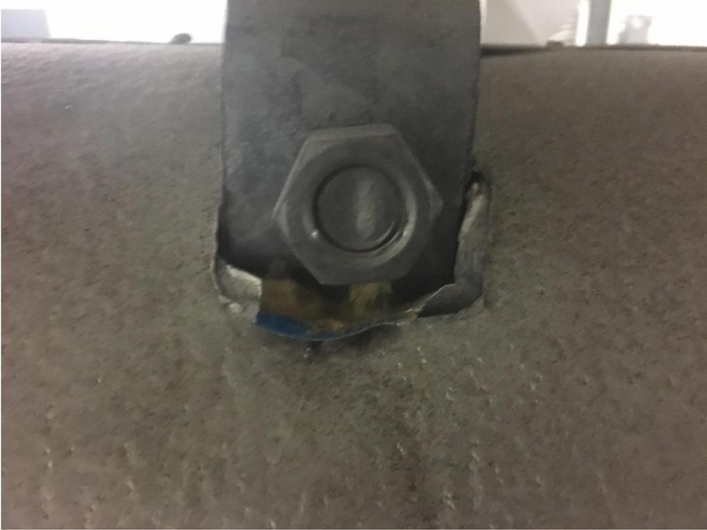
*Figure 21 – Observed Fiberglass Insulation around pipe, no need to sample*
