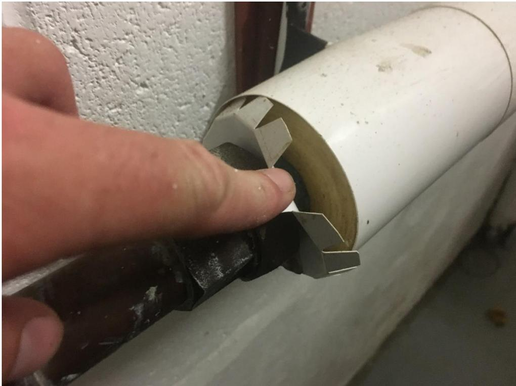
*Figure 44 – Observed Fiberglass Insulation, no need to sample*
