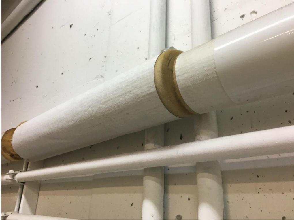
Figure 17 – Observed Fiberglass Insulation, no need to sample
