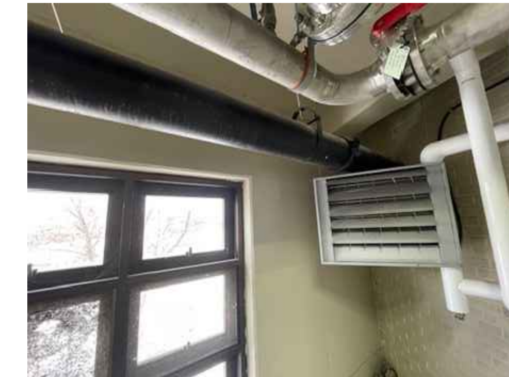
PHOTO No.2 EXISTING DIGESTER #2 GRAVITY TRANSFER
