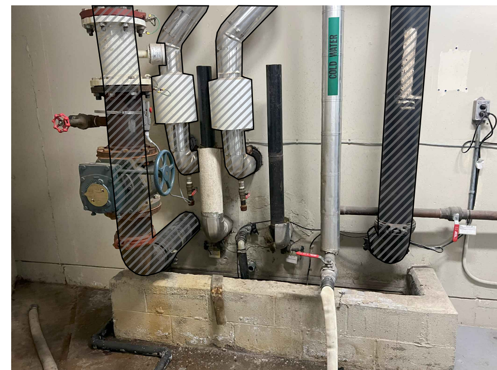
PHOTO No.2 EXISTING DIGESTER SLUDGE INLET/HYDRONIC INLET SCALE: N.T.S.
