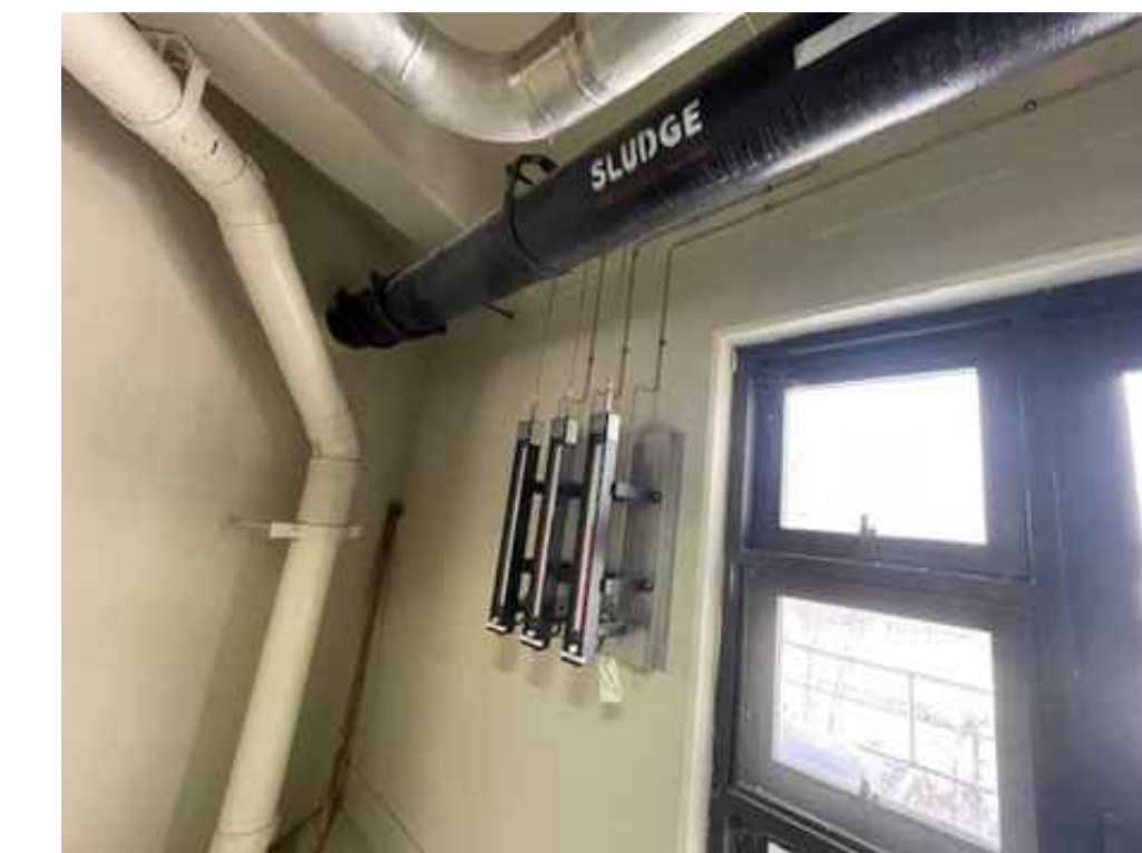
PHOTO No.1 EXISTING DIGESTER #3 GRAVITY TRANSFER
