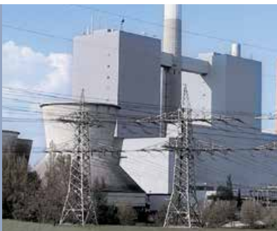
Indispensable for power plant technology
