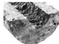
Diamond cored hole with roughening
