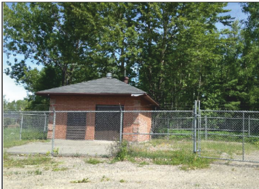
Photo 11: Hudson Rd. Lift Station – exterior brown paint located on vent (14 000 µg/g or 1.4% lead by dry weight).
