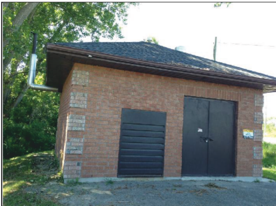
Photo 6: Kingsway Lift Station - Exterior
