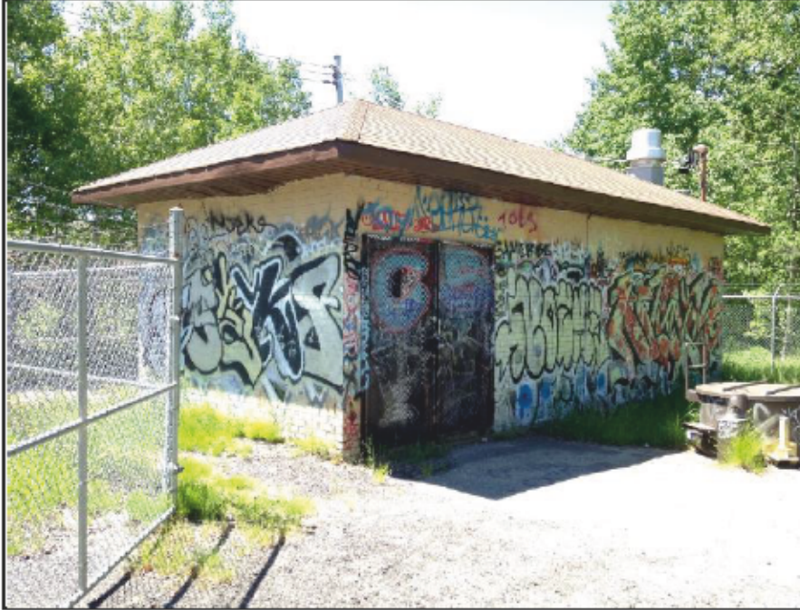
Photo 1: Bancroft Drive Lift Station – Paint damaged by graffiti.
