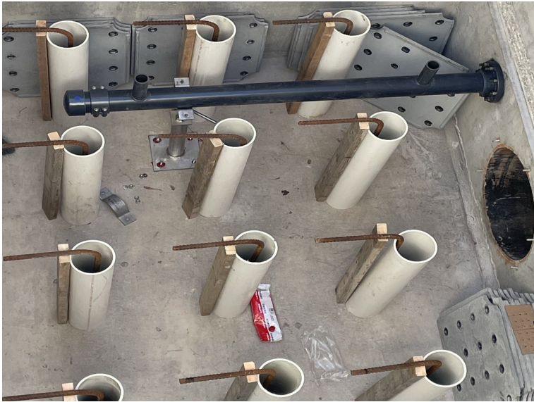
Installation of Starter Bars
