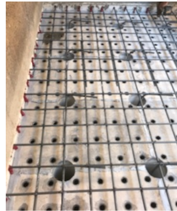
Completed Reinforcement (Tied into Walls with Adhesive Anchorage)
