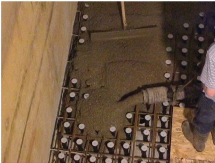
Placing of Concrete to Form 6" Slab
