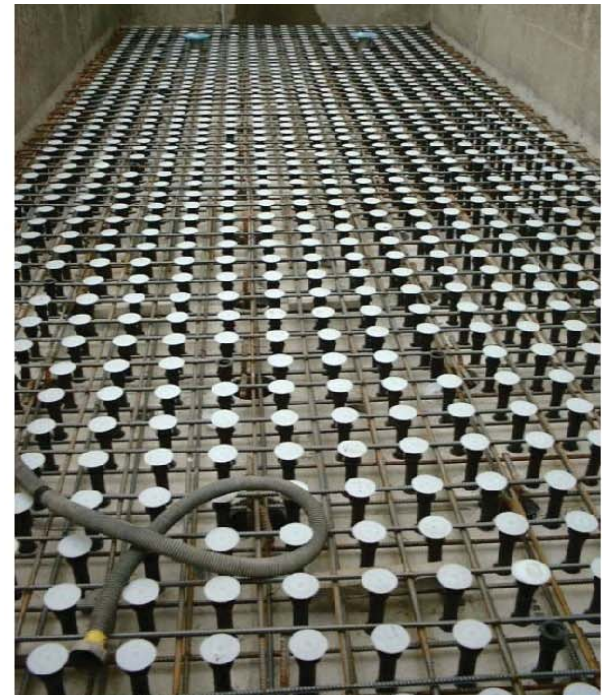
Install of Sleeves with Caps
