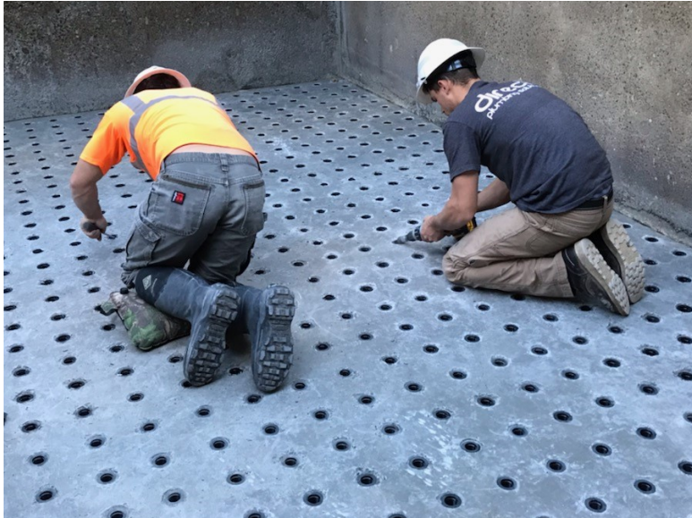
Clean Up of Concrete
