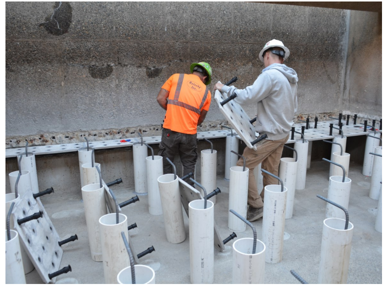
Pedestals with Starter Bars
