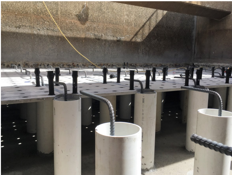
Panels in Place on Pedestals
