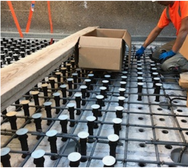
Install of Sleeves with Caps
