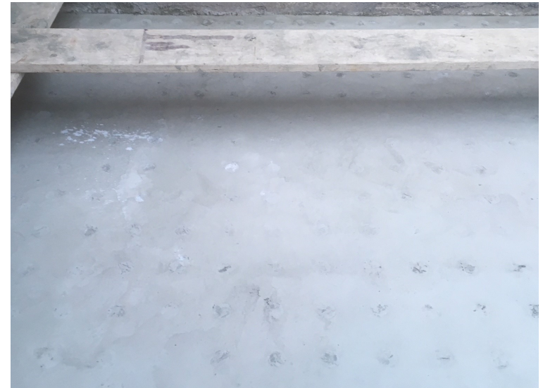
Concrete in Place & Curing
