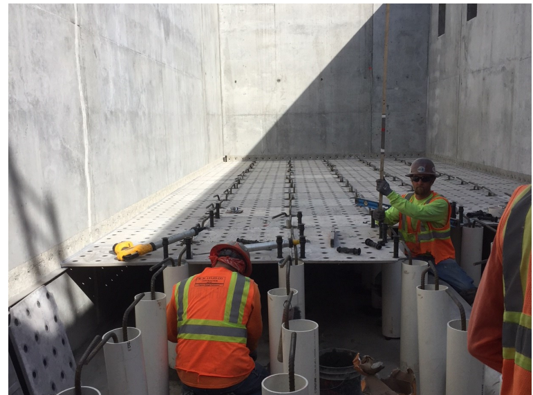
Verifying Panels are Level
