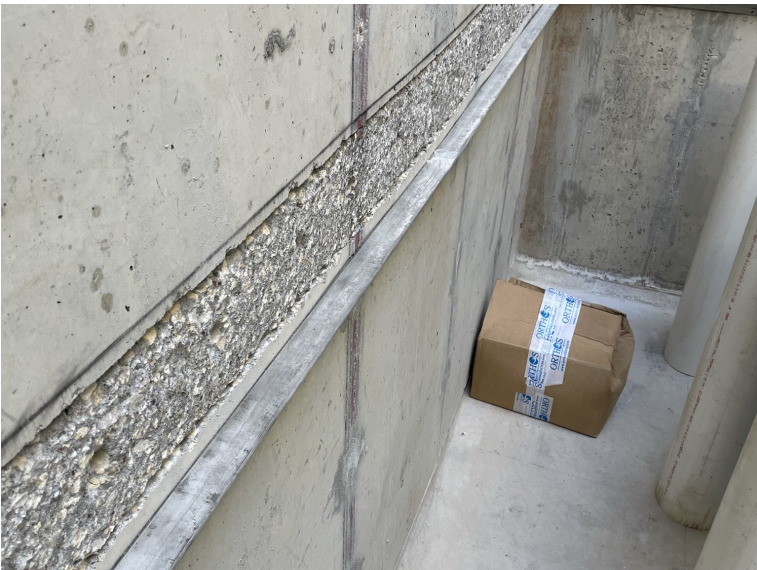
Installed 316 SS Angle Support
