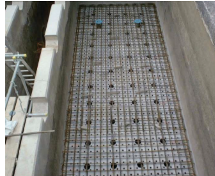
Panels and Reinforcement Completed for Filter Basin
