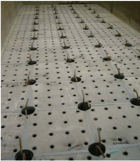
Panels Secured in Place with Mastic
