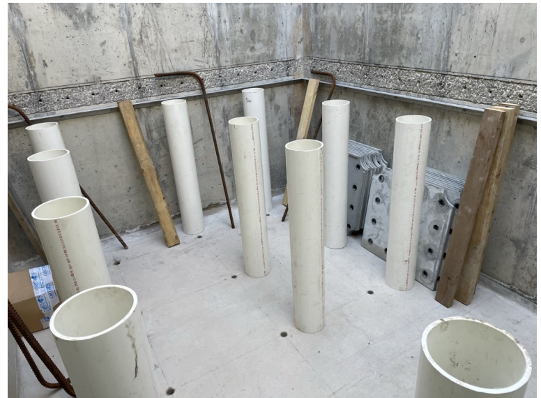
Starter Bar Holes & Dowel Holes
