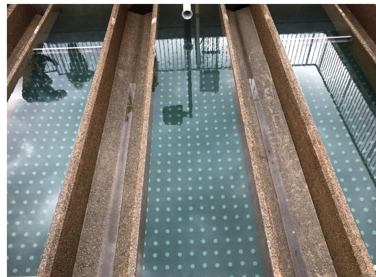
Nozzle Install Pre Media Placement
