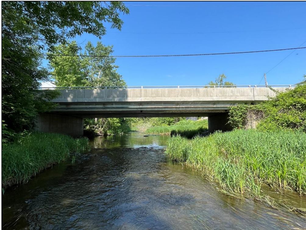
Photo 2 – East elevation of structure.
