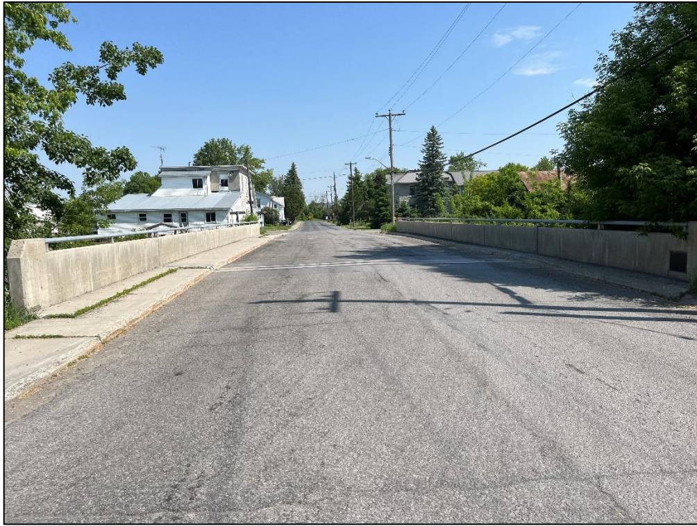
Photo 1 – Deck cross-section from south approach looking north.
