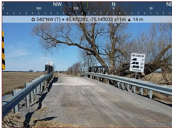
Site Photograph 5 – Bridge, looking north. Single large tree adjacent to bridge.
