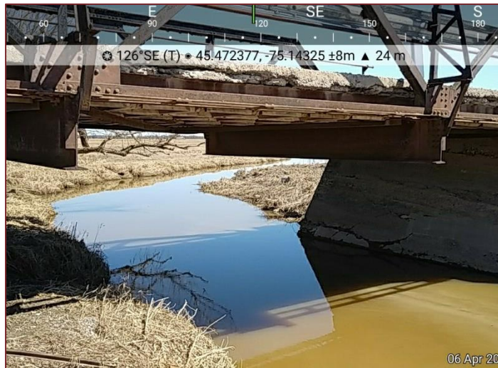
Site Photograph 3 – Upstream aspect of bridge.
