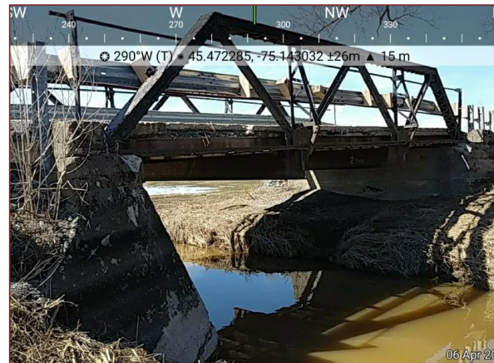
Site Photograph 4 – Downstream aspect of bridge.
