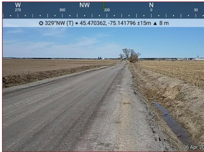
Site Photograph 1 – Southern extent of study area, looking north towards bridge.
